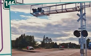
new railroad crossing 8th Street / nuevo cruce de ferrocarril calle 8th
