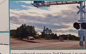
new railroad crossing 3rd Street / nuevo cruce de ferrocarril calle 3rd
